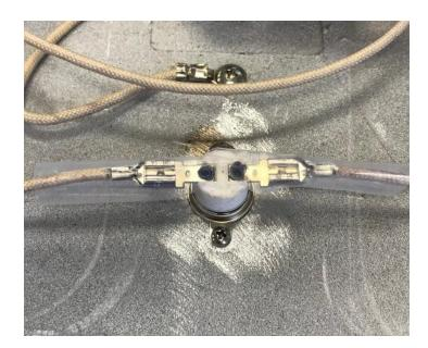
Reattach the heater wire ends making sure to install the included heat shrink tubes.
